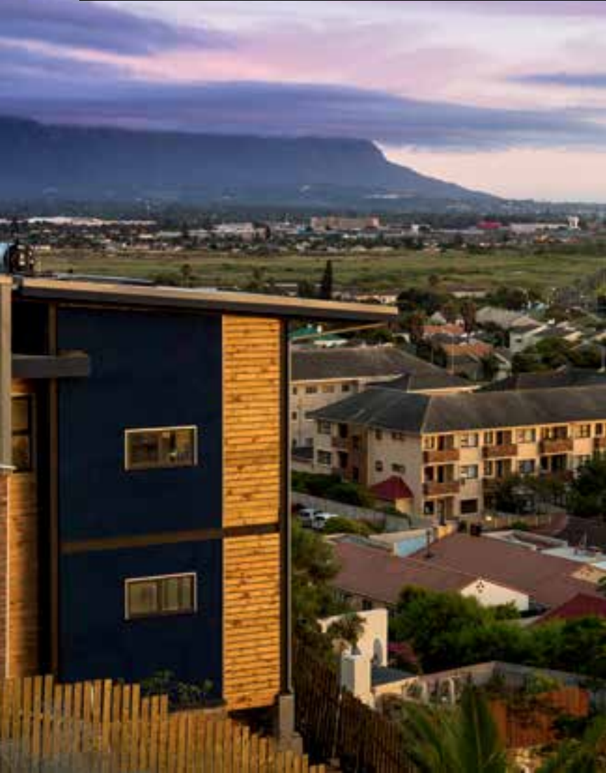
The house was conceived as a series of staggered levels flowing down the site. The south facade is clad with Nutec board and corrugated sheeting, painted navy blue, lending the house a nautical feel.
